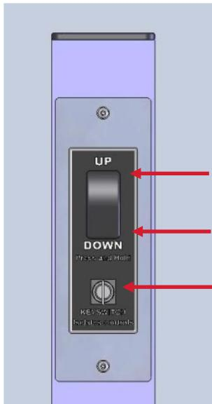
Press and hold the top of the rocker switch to call or send the lift up.
